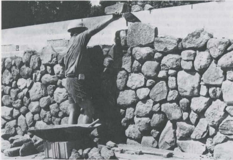
Jim Milano of Milano Masonry at work on a wall of the new museum building. Photo by Michael D'Amore
