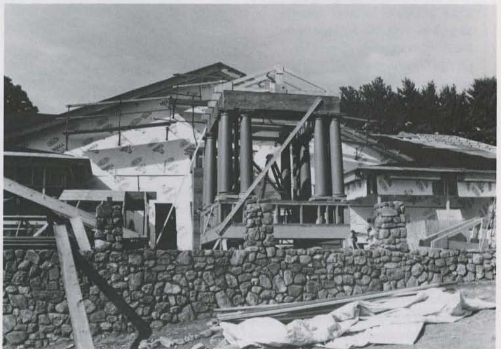
Cupola assembly on terrace. The cupola was installed on the roof on November 8. Pictures in next Portfolio .
