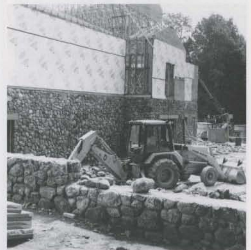
Clean-up after masonry work is complete
