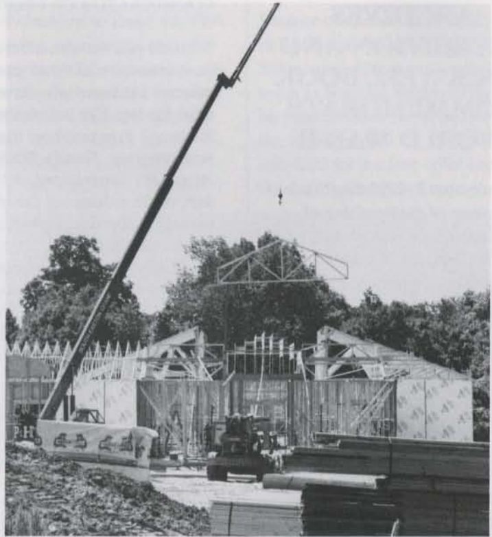
A roof truss going up
