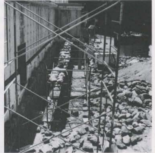
Installation of west wall masonry
